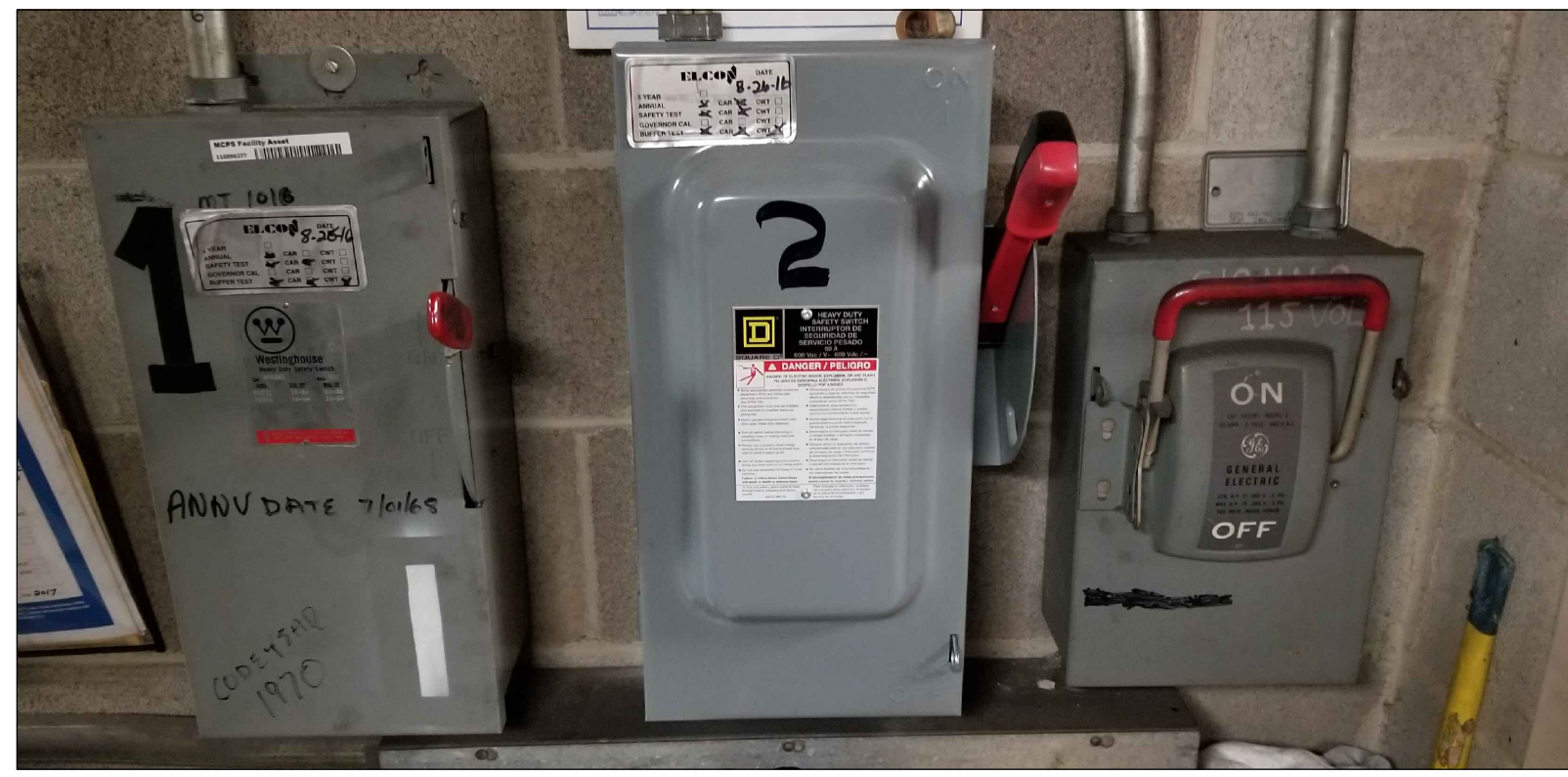
EX. ELEVATOR DISCONNECTS SCALE: NOT TO SCALE
